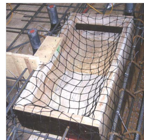
Pour-in-place net protection
