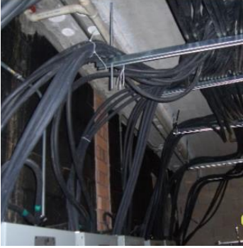
Temporary cable due to failure of existing busway
