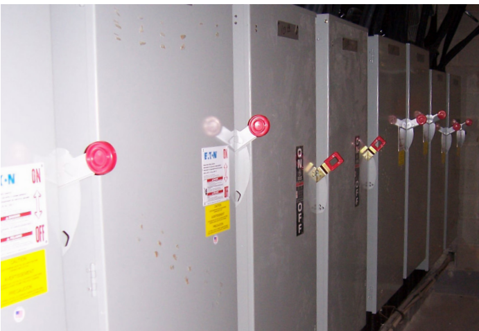
Temporary disconnects to each floor as a result of busway failure. As depicted in the temporary repair photos, emergency power restoration due to busway failure initially took five days. Entire busway had to be replaced due to severe arcing and destruction with additional downtime for permanent repair.
