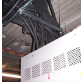
Temporary cables to each floor of condominium due to busway failure
